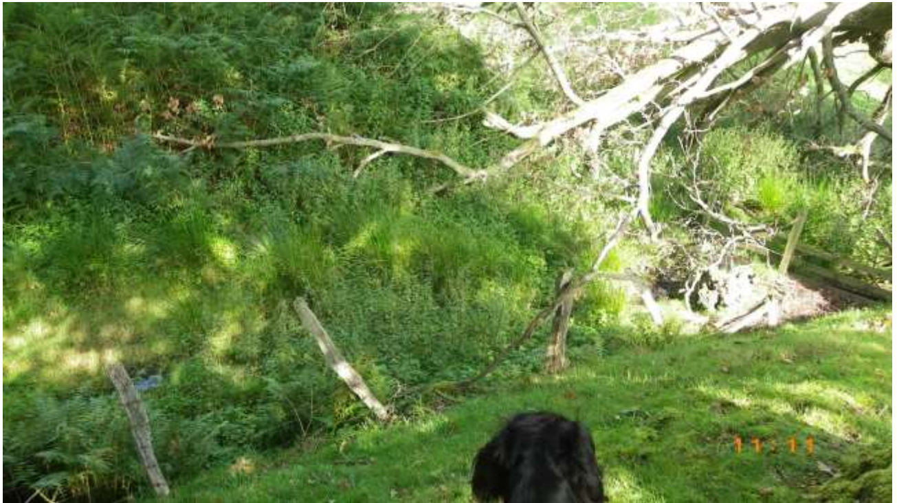
Photo 269 & Cpt19a fence to the south no longer stock proof
