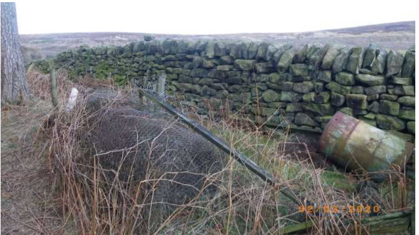
Photo 53 Cpt3a old fencing stacked for removal
