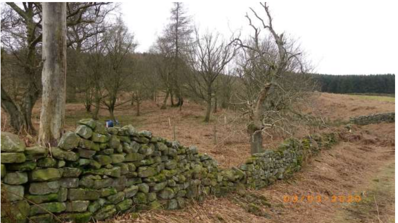
Photo 34 Cpt 2a the eastern boundary wall
