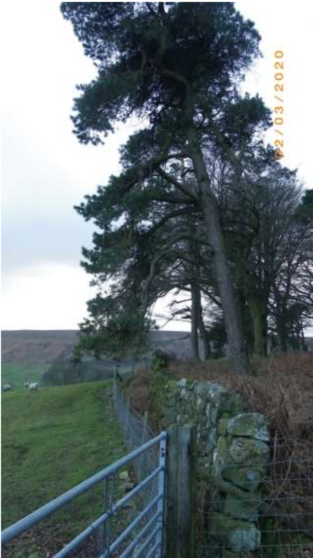
Photo 70 the southern boundary wall of cpt5a is stock fenced to the field side
