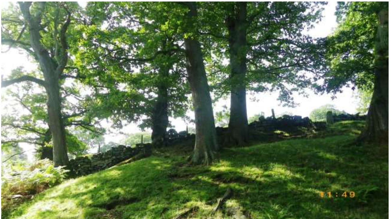
Photo 274 Cpt20a boundary wall with fencing to the s/w boundary; not secure
