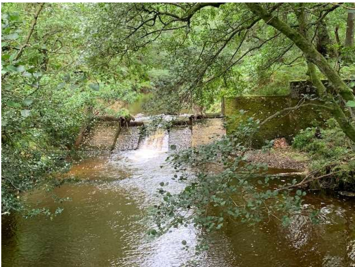
Photo 312 The weir up stream of the footbridge across Hodge Beck
