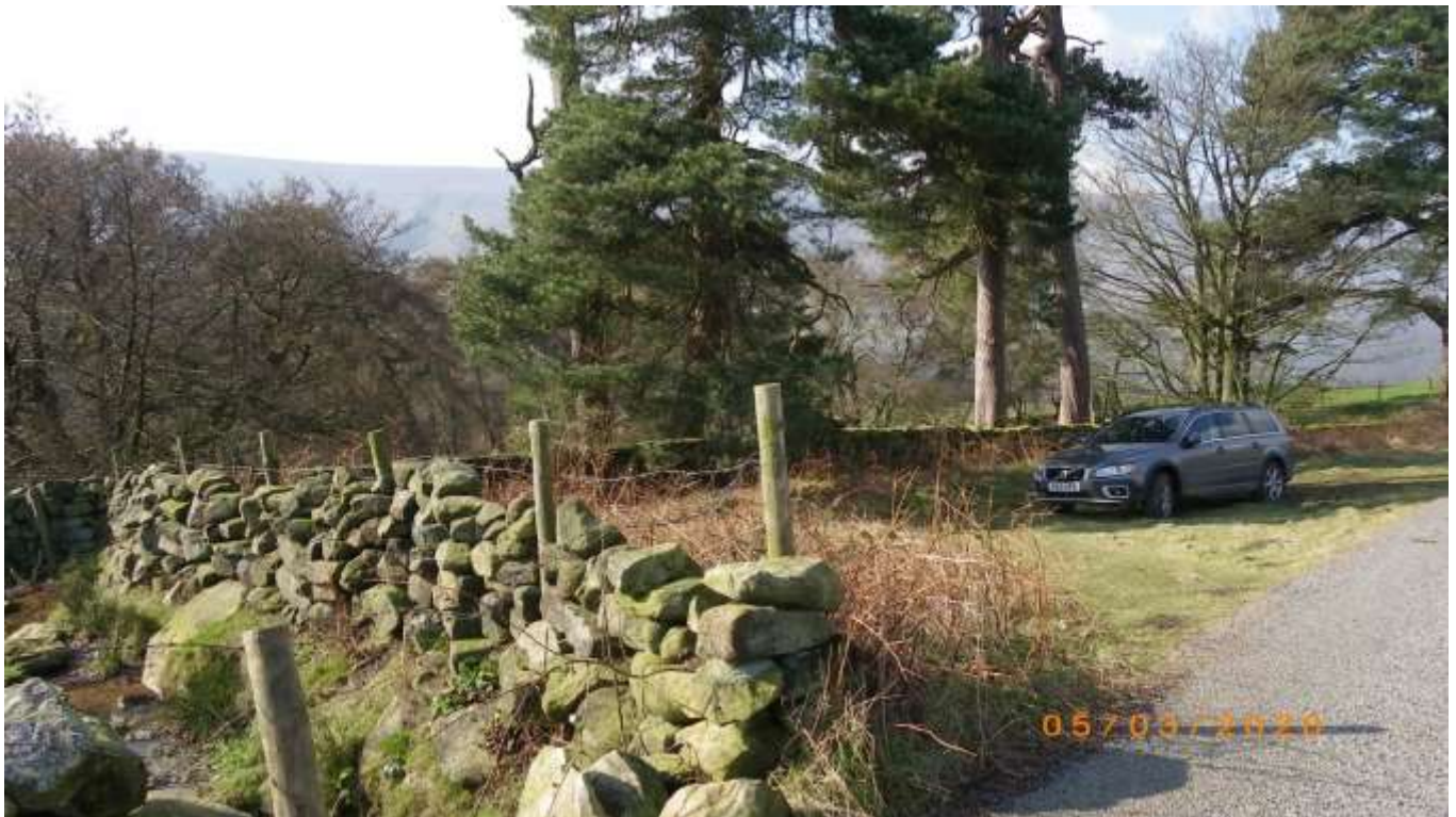
Photo 430 Cpt26 Sonley Woodland the n/e boundary to Daleside Road
