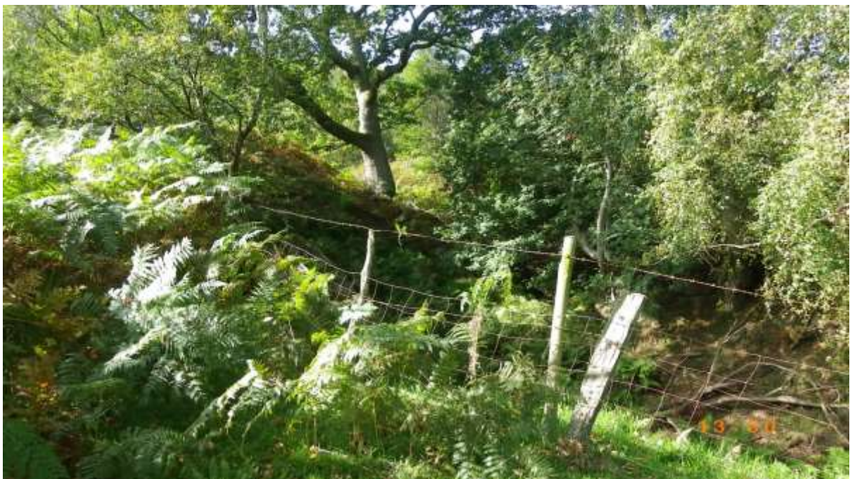
Photo 261 Cpt17c poor fence along the southern boundary.
