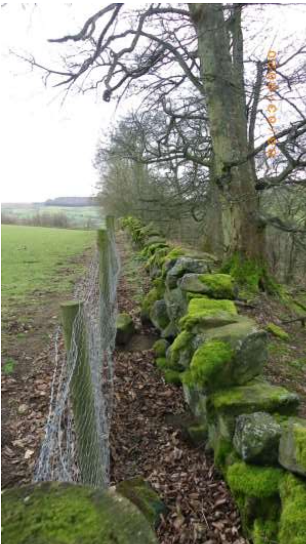
Photo 88 Cpt7a eastern boundary, old wall and stock fence to field side
