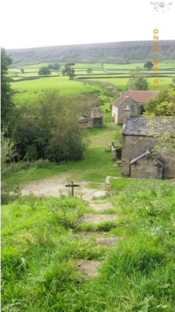
Photo 139 Bransdale Mill buildings and note PROW sign for footpaths and bridleways.
