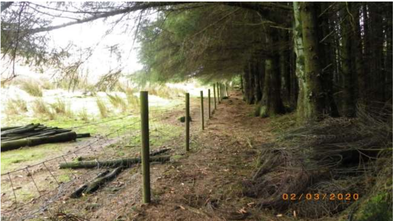
Photo 64 Cpt4b stock fence to the westerly boundary
