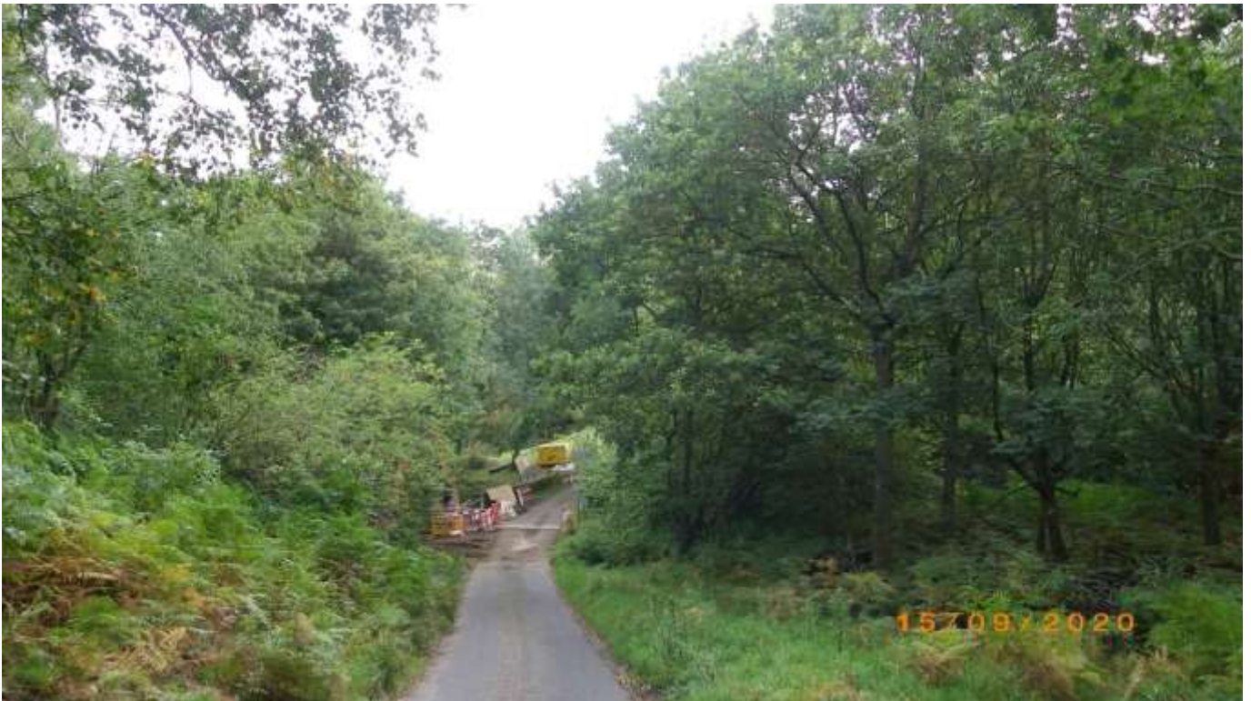
Photo 180 bridge over Hodge beck with cpt11 to the north (right) and cpt12 to the south
