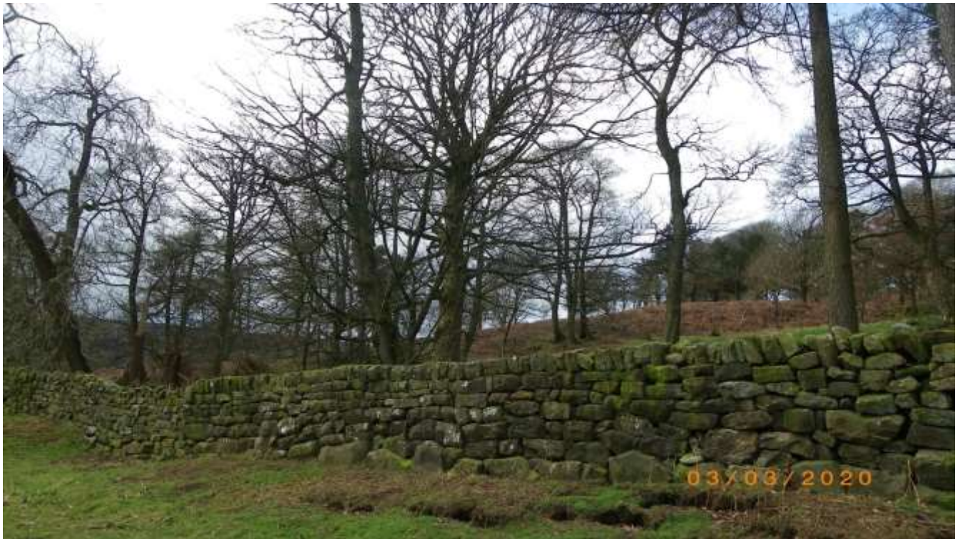
Photo 49 south east boundary to Heater Plantation good condition
