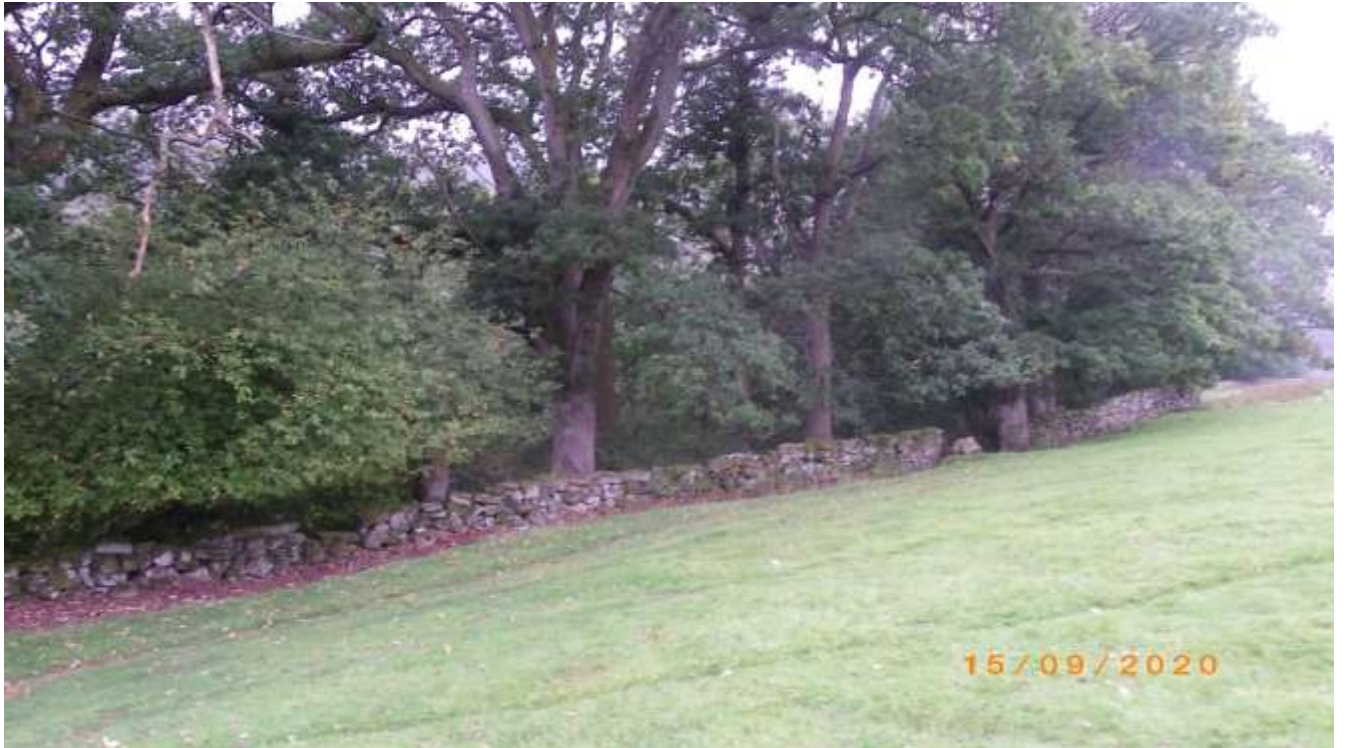
Photo 402 & 403 Cpt22a Low Wood boundary wall collapsed in several places to the north west and the wood is grazed in parts
