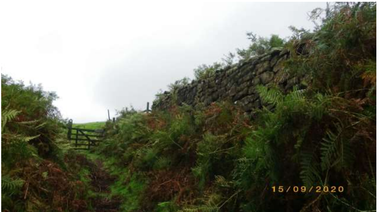
Photo 304 boundary wall to the south west towards Stork House
