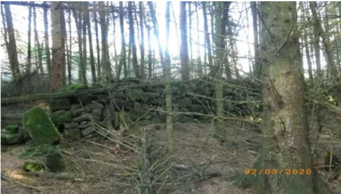
Photo 7 Cpt1a old wall to eastern boundary with Forest England
